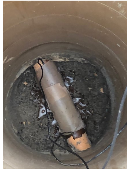
Figure 4- Wax coating applied through keyhole
