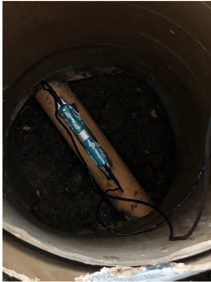
Figure 3- Keyhole install on a 2" gas line
